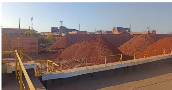
Figure 1 – The charging yard on the PAP
