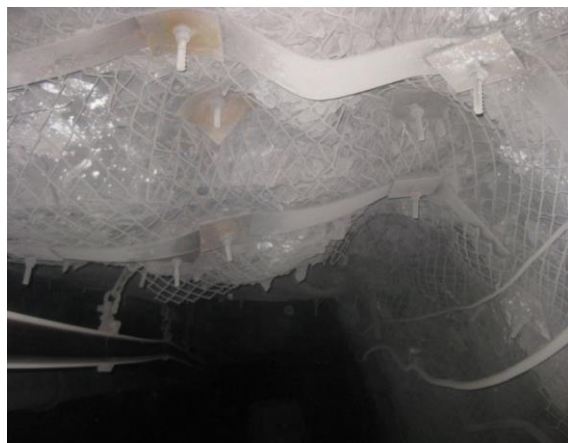
Figure 6 – Deformations of contours of belt entry 231k 19 -s of Abaiskaya mine, Karaganda coal basin
